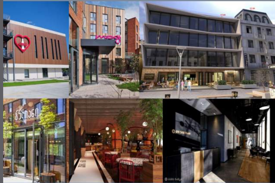
JSC. "Medical Corporation Evex" office complex (MEP)
